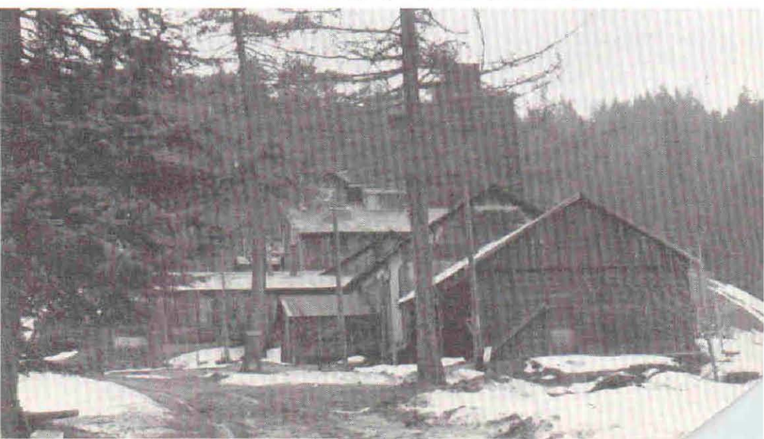
Mill building at the Sierra zinc property, near Colville, Wash.
