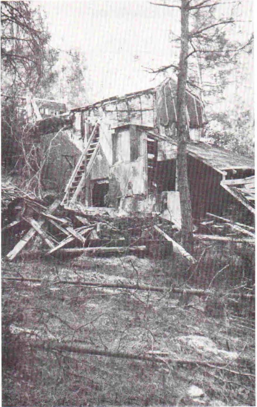
Decaying mill building north of Bossburg, Wash.
