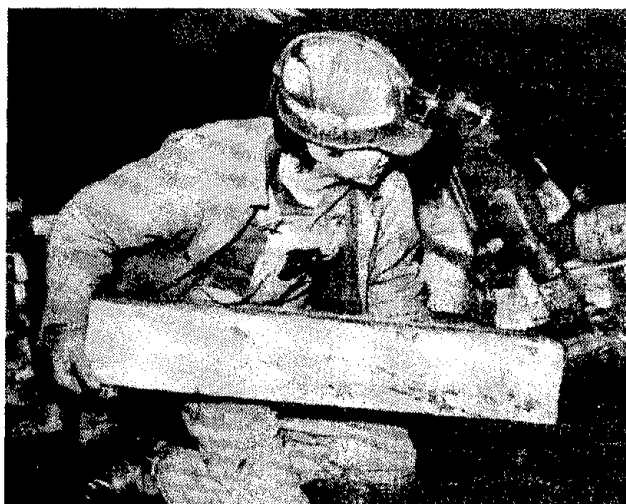
Figure 1.—Low-seam coal miner ready to throw a 6- by 6-in cribbing block, weighing approximately 35 lb. The kneeling posture imposes considerable torsional stress on the lower back because the workers cannot easily reposition their bodies.
