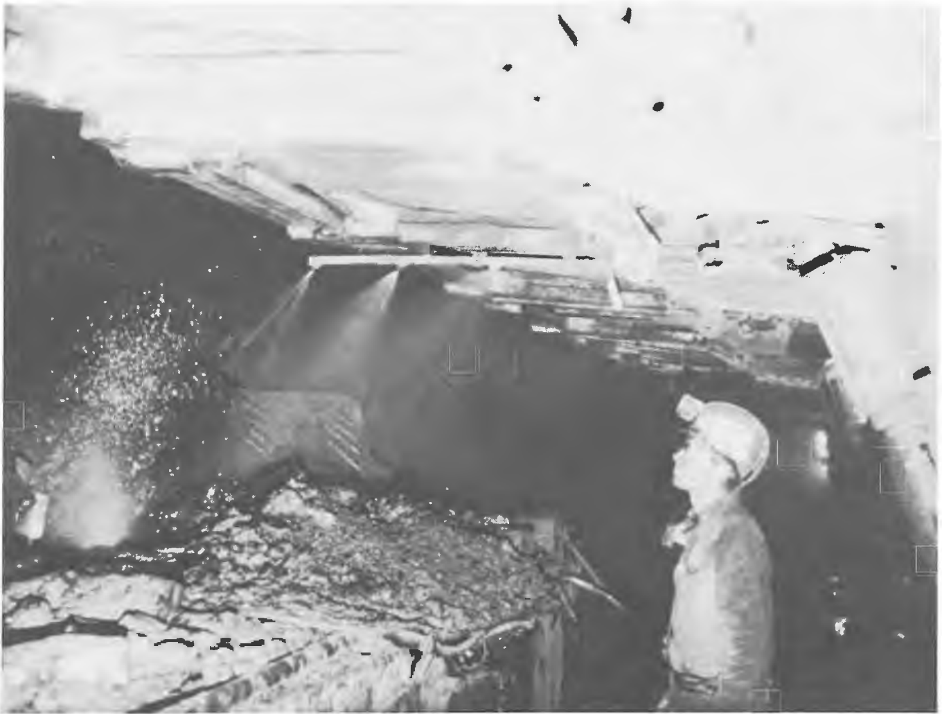
FIGURE 8. - Spray manifold located on support canopy.
