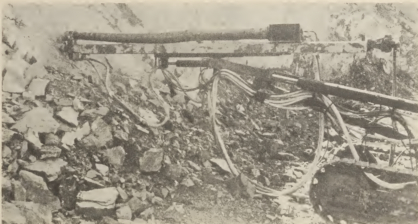
FIGURE 38. - Redesigned, noise-controlled jumbo drill at start of hole.
