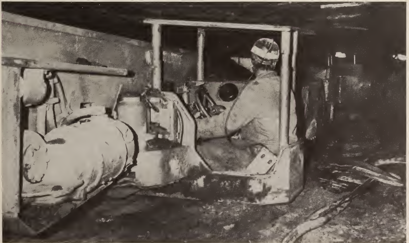
FIGURE 8. - Side-saddle tram compartment on end-driven shuttle car.
