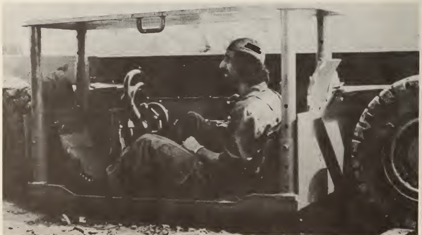
FIGURE 9. - Prototype floating cab on center-driven shuttle car.
