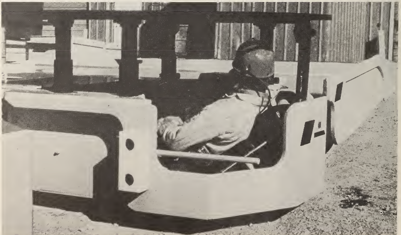
FIGURE 9. - Operator's deck on scoop extended beyond side of machine.
