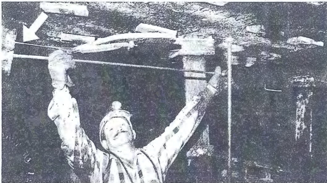
Figure 1.—Antenna used by bolting machine operators to gauge the distance between rows of bolts. Arrow indicates antenna. (Courtesy Jerry Taylor, Ohio Valley Coal Co., Powhatan No. 6 Mine.)
