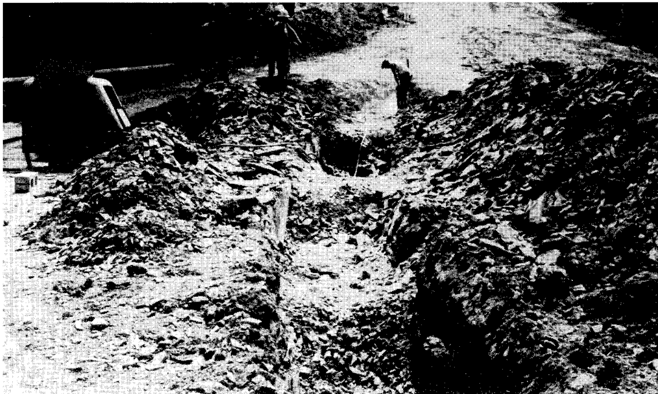
FIGURE A-4. - Cutting utility trench in solid rock near the fanhouse.
