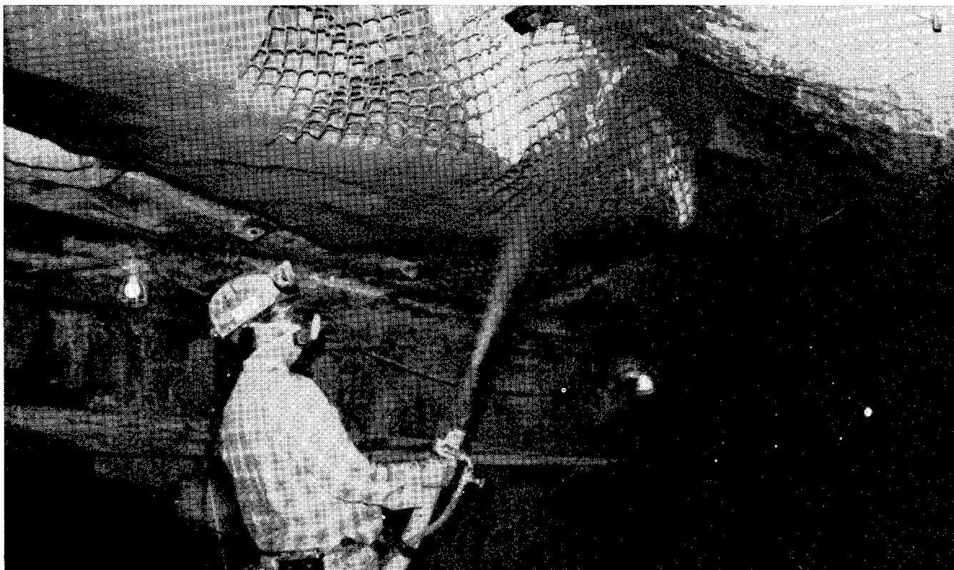
FIGURE A-16. - Installing gunite (fibrous) on a fault in B-drift.
