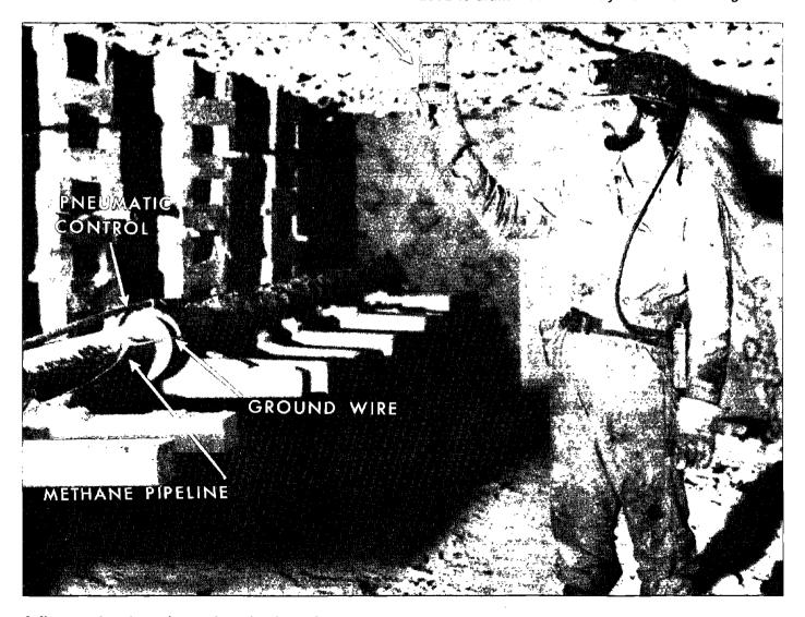
A flame safety lamp is used to check methane levels near an underground methane pipeline. If the pneumatic control line on top of the pipe is
