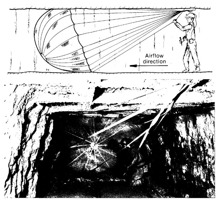
Straps hooked on a roof bolt or other projection hold the parachute stopping in place. Air pressure across the parachute stopping forces it against the mine roof, walls, and floors, forming a good air seal.
