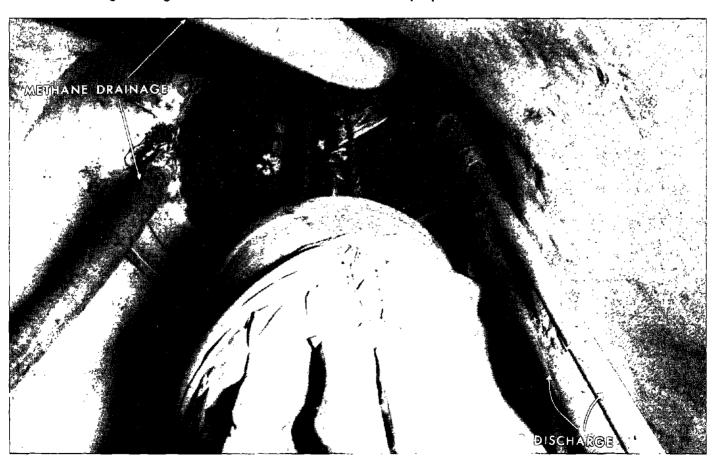
Methane drainage through shafts. Methane is carried to the surface through 4-inch hoses behind the 4-foot-diameter casing, while smaller pipes remove water. Bucket in center is used to transport workers and equipment between the surface and the bottom of the shaft.
