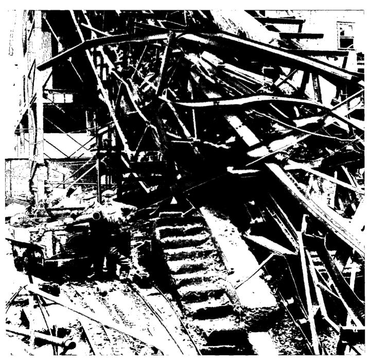
The force of an underground explosion wrecked the tipple at the Kimlock Mine, Parnassas, Pa., in 1929. (Photo from Bureau of Mines files.)
