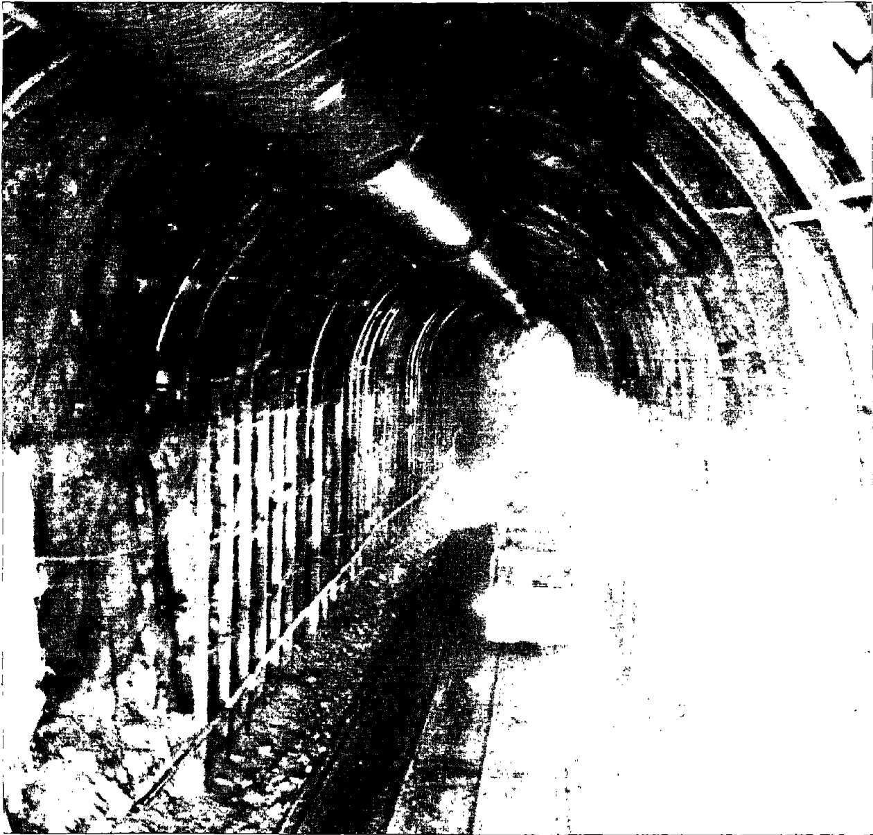
FIGURE 16. - Steel support in north heading.
