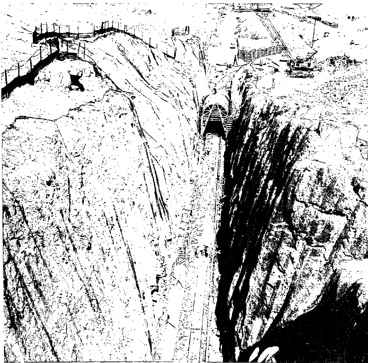
FIGURE 35. - Typical concrete formwork section at north portal.
