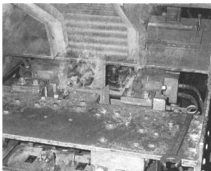
FIGURE 7. Sparks and fire on top of the ERH, probably due to heating of oil residuals.
