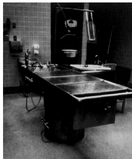
FIGURE 1. Downdraft ventilation table showing the pedestal base and drainboard consisting of three movable perforated panels.
