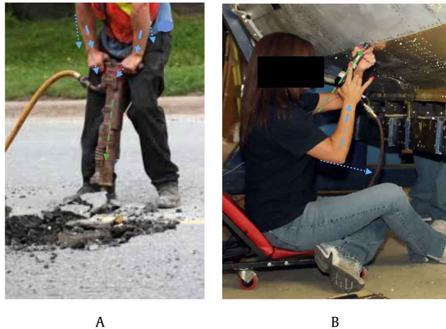
Fig. 2. Examples of tool operations and three coordinate systems. (A) Jack hammer used in repairing a road (Adapted from www.hsa.ie/eng/Topics/Physical_Agents/ ). (B) Rivet hammer used in repairing an air plane frame. The green dashed arrow (--->) represents the z axis (tool action direction) of the tool coordinate system, blue dashed-dotted arrow (-.-.->) the z axis of an anatomical (forearm) coordinate system, and the blue dotted arrow (.....>) the z axis of a local skin coordinate system.
