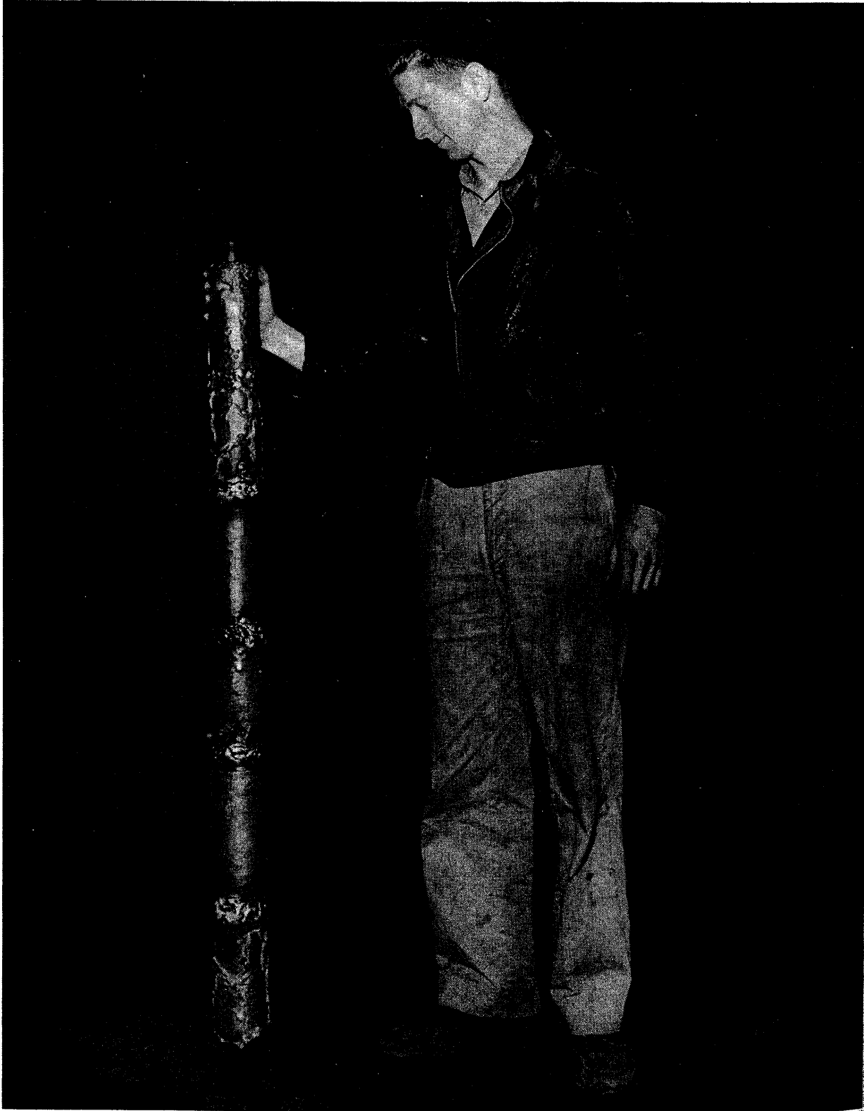
FIGURE 6. - Consumable Electrode Formed by Welding Molybdenum Reguli Together.
