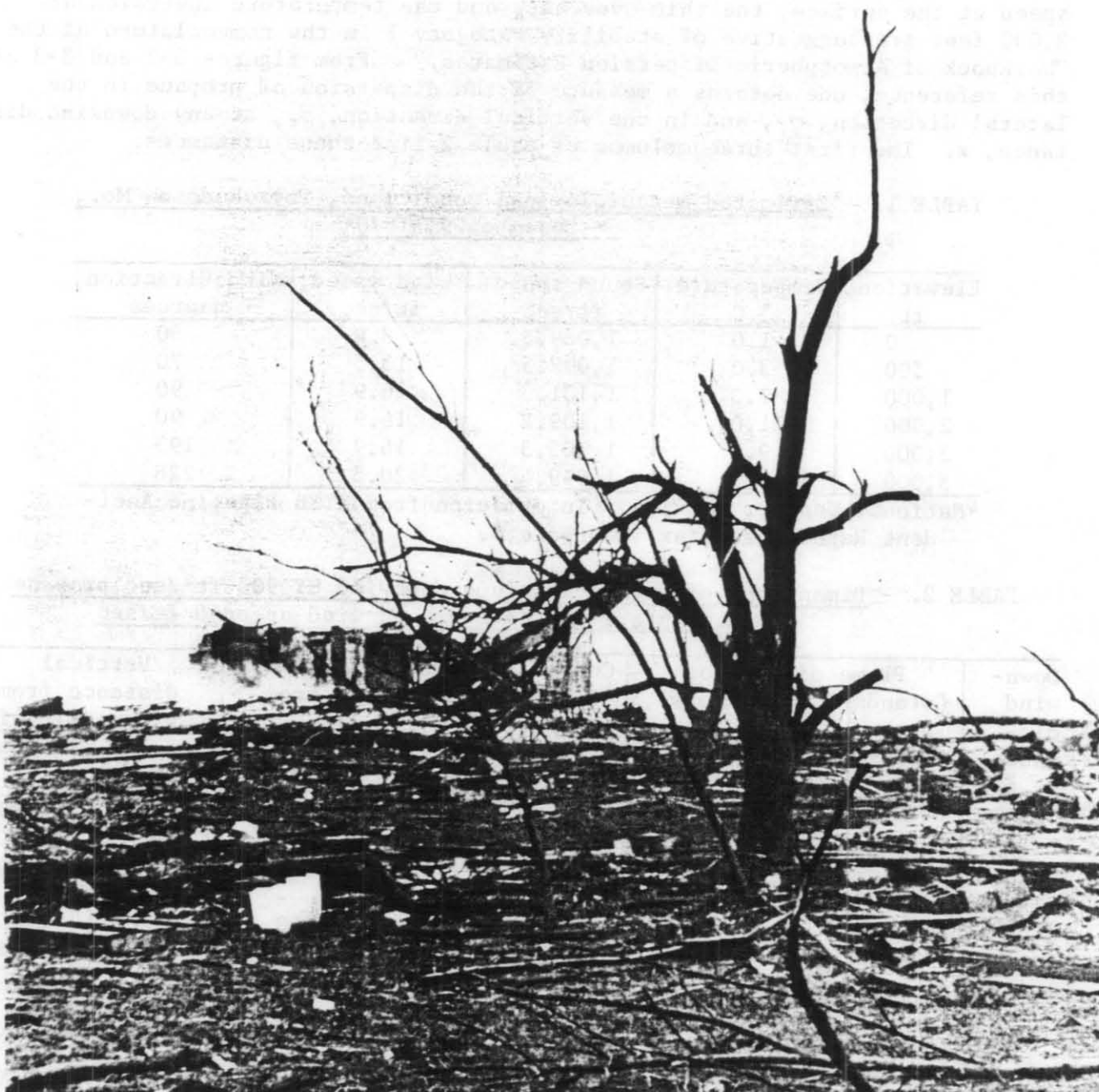
FIGURE 10. - Aftermath of detonation and firestorm, near presumed point of ignition.
