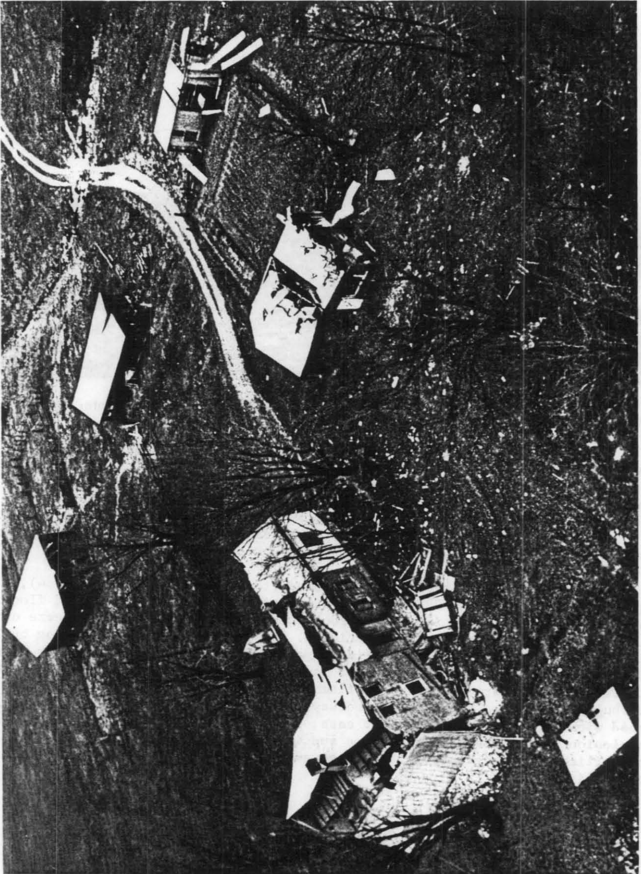
FIGURE 8. - Damage to Stotko farm, about 2,000 feet southeast of center of blast.
