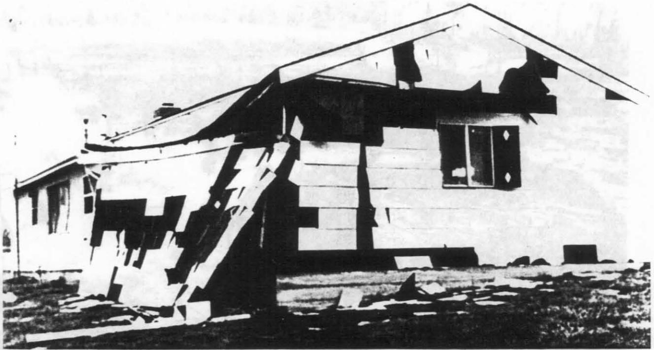
FIGURE 5. - Damage to Hubenthal home, about 1,500 feet north-northwest of presumed center of blast.
