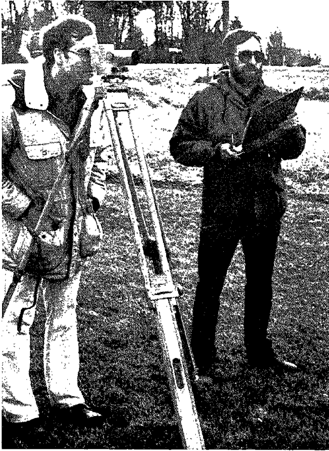
Figure 12.—Survey crew performing level-loop analysis.
