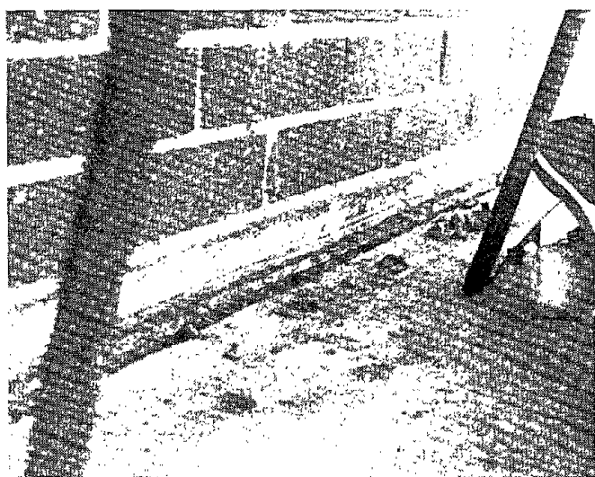
Figure 26.—Junction of north wall and patio of house 201 showing evidence of settlement.
