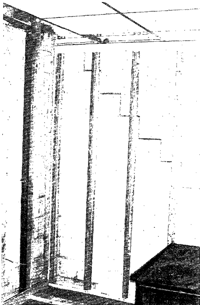
Figure 24.—Basement block wall crack on east wall of house 201.
