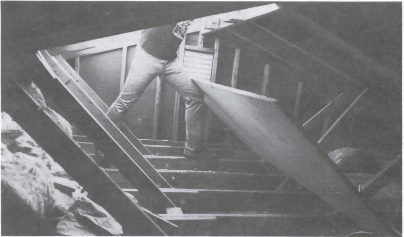
FIGURE 9. • Roof joist preparation for mechanical shaker installation.
