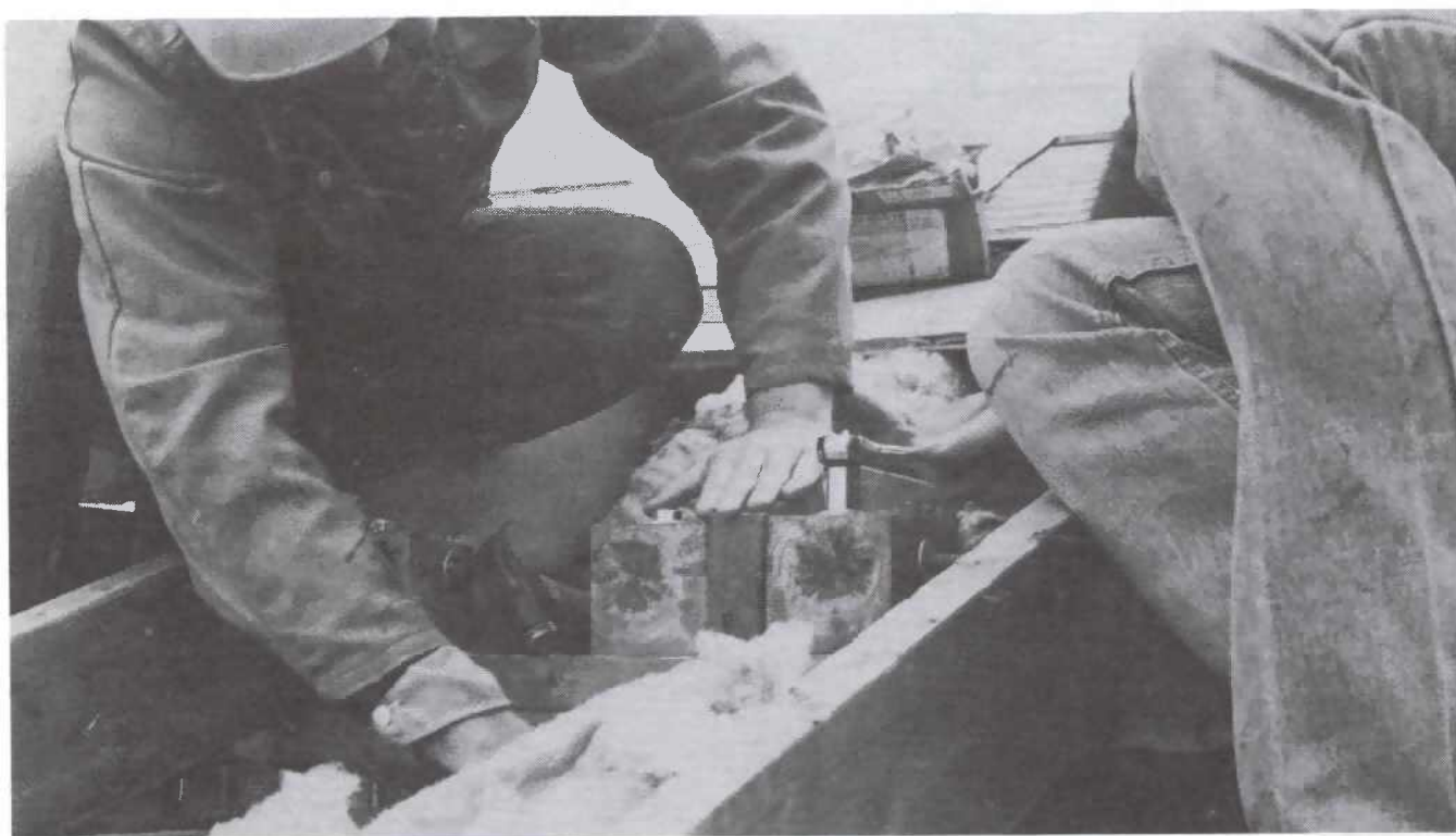
FIGURE 12. - Ceiling joists being bolted to wall studs.
