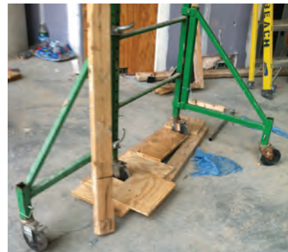
Figure 3: Improperly secured base on mobile scaffolding
