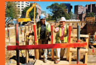
AUGUST Early construction: Sheeting and shoring process
