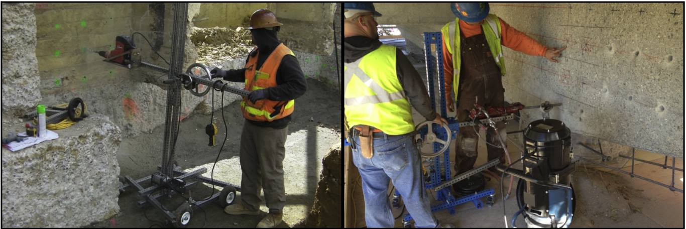
Fig. 2. Construction workers using early versions of the universal rig with an electric hammer drill on a stadium upgrade (left) and a pneumatic rock drill on a train tower (right).
