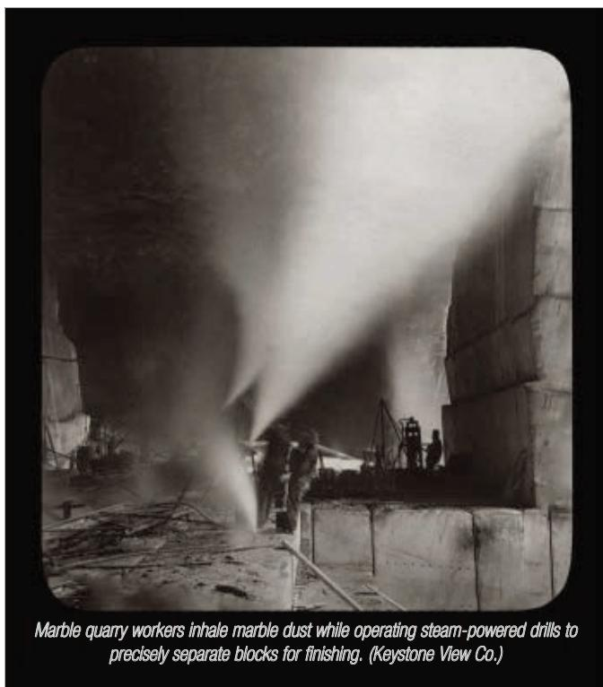
Marble quarry workers inhale marble dust while operating steam-powered drills to precisely separate blocks for finishing. (Keystone View Co.)
