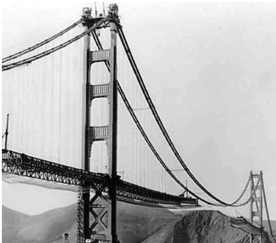
Golden Gate Bridge deck hung from cables while under construction, photographic print: b&w. 20 x 21 cm. (7 3/4 x 8 1/4 in.) 1965
