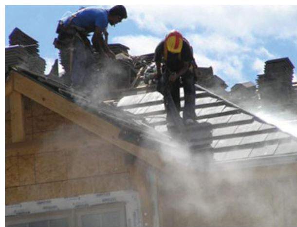
FIGURE 4. Workers using a leaf blower to clean dust from tiles. (color figure available online)
