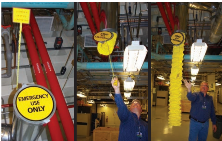
Figure 2. PtD hazardous chemical containment system at Birck Nanotechnology Center (BNC). Hatches such as the one shown here are strategically placed throughout the BNC subfab area. These hatches are connected to a duct system containing elephant trunks that workers can use to exhaust the accidental release of hazardous chemicals or gases.
