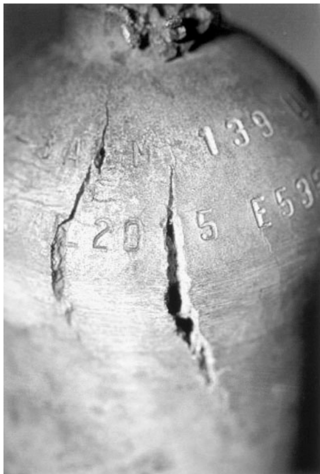
FIGURE 2. Compromised oxygen cylinder from Case no. 2.
