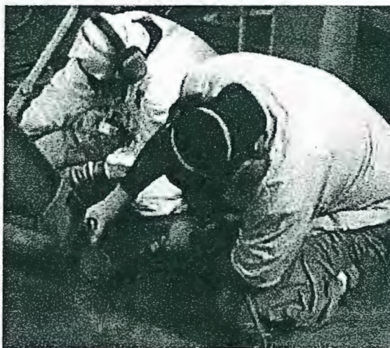
Figure 10 - Deck Scraping
