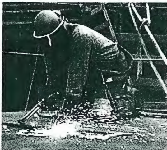
Figure 8 - Torch Cutting on Deck
