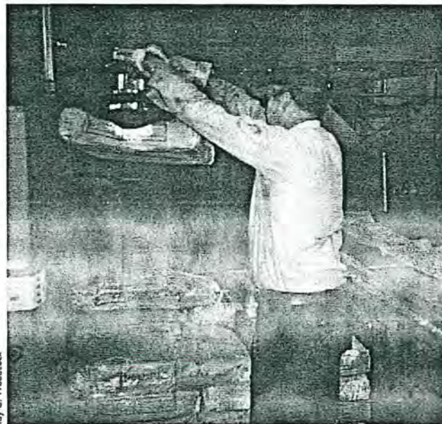
Figure 80.10 • A vacuum lift carries bags to the charging conveyor for a Banbury mixer, eliminating back strain from manual handling.
