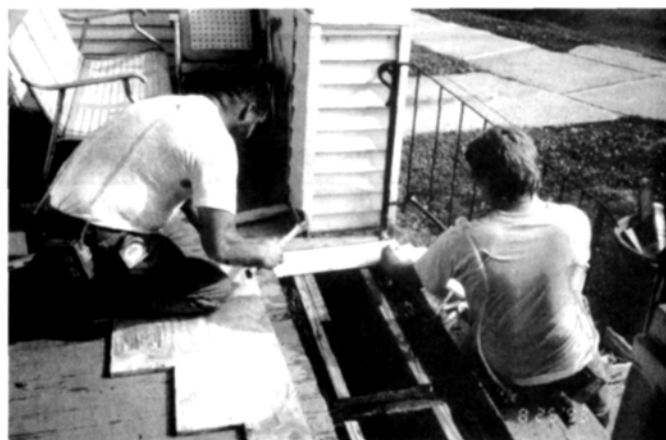
FIGURE 3. Workers repairing a painted porch floor.
