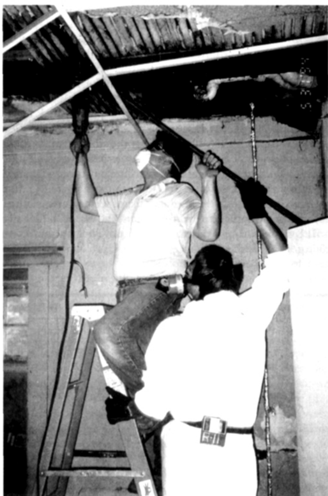
FIGURE 2. Workers manually demolishing a deteriorated plaster ceiling.
