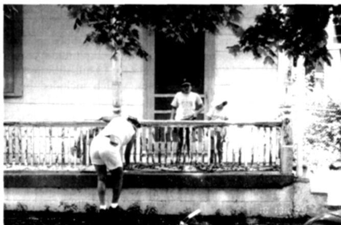
FIGURE 1. Worker dry scraping exterior paint during home painting event.
