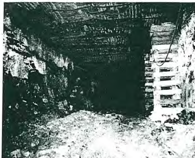
Figure 9 — Condition of 1 st entry after failure.
