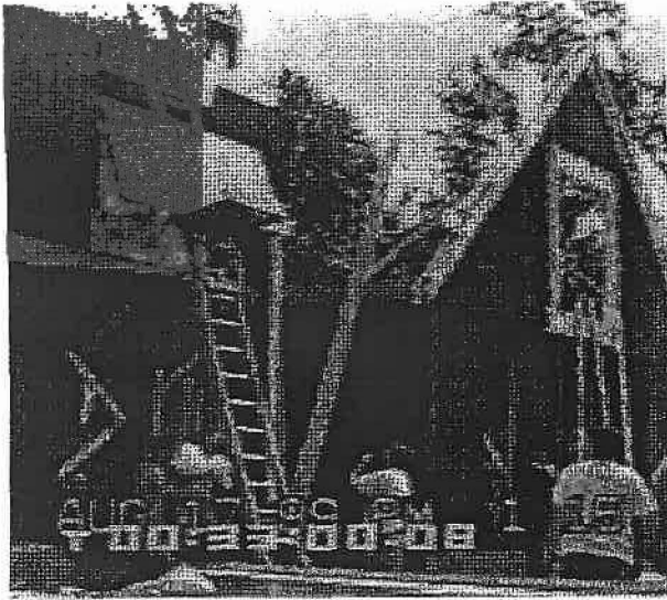
Figure 3. Vertical material lift to move materials to the second and third stories of a structure
