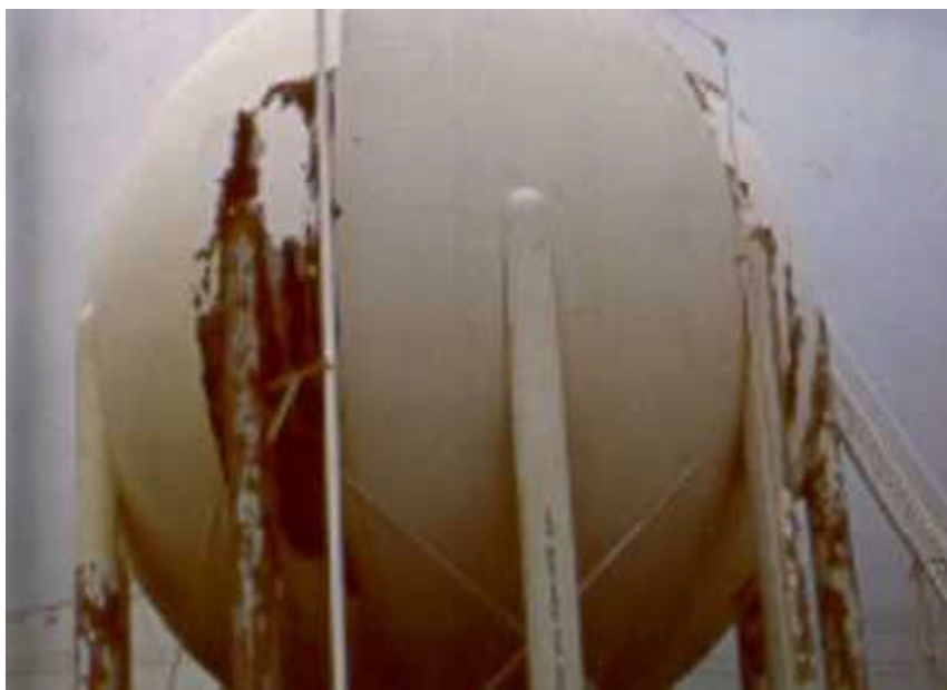
Peeling lead paint on a chemical tank.
