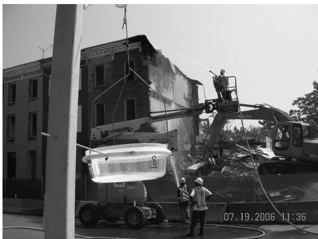
Photo 5. Extensive dust suppression used at a housing demolition site in Baltimore, with simultaneous water application to roof and to debris pile below. Lead dust fall sampler shown in foreground. Source: East Baltimore Development Initiative
