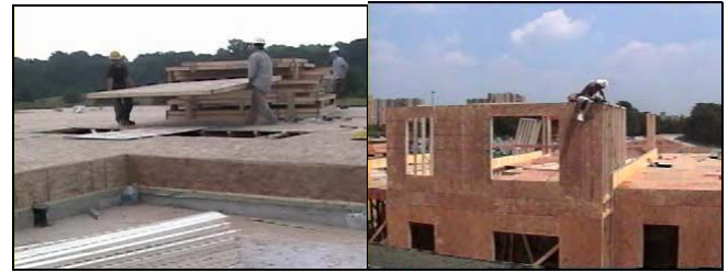
Figure 1. Samples of video captured incidents at the residential construction sites. Carrying over uncovered holes on the work site (left) and fixing on the top without a life line (right)
