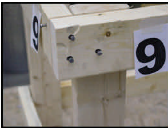
Figure 6. Overlap Mid and Top Rails
