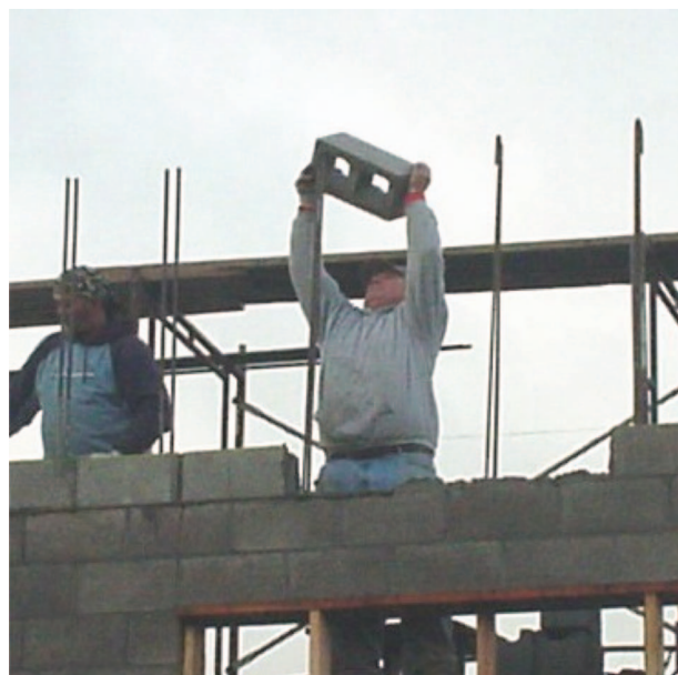
Figure 2. Bricklayer placing CMU block onto vertical rebar.
