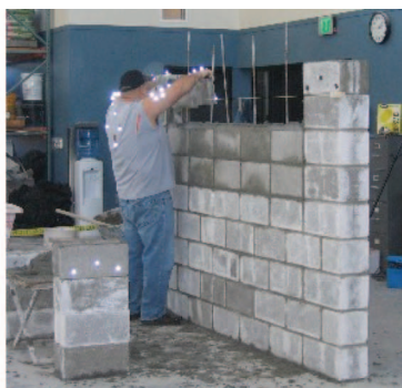
(a) Placing conventional CMU
