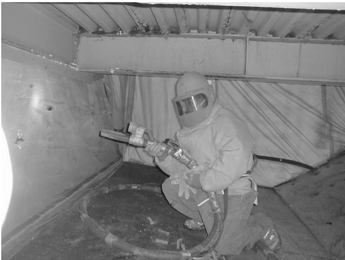
FIGURE 1. Abrasive blaster wearing Type CE supplied-air respirator in containment area (Photo by Norman Zuckerman)
