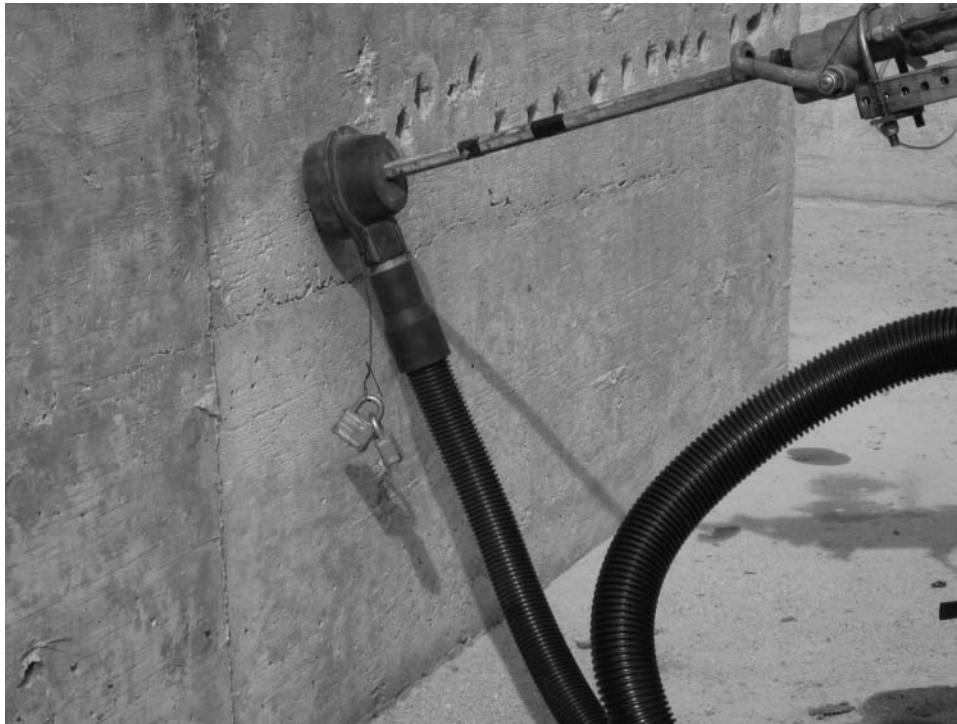
FIGURE 3. Dust capture shroud functioning while drilling. The locks were added to provide weight to the shroud so that it would slide toward the hole while drilling.
