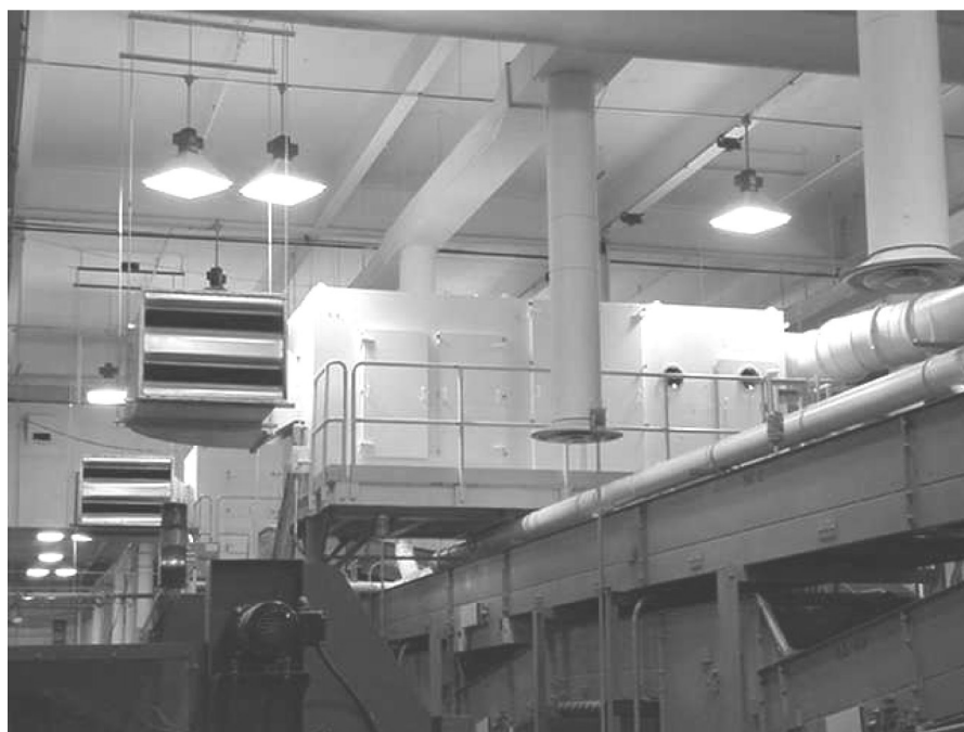
FIGURE 5. Part of the ventilation and filtration system installed on a USPS 010 Culling System. The large white filter/fan housing suspended above a Loose-Mail Distribution System is one of the 18,000 cfm (8.5 m 3 /sec) units tested as part of this study.
