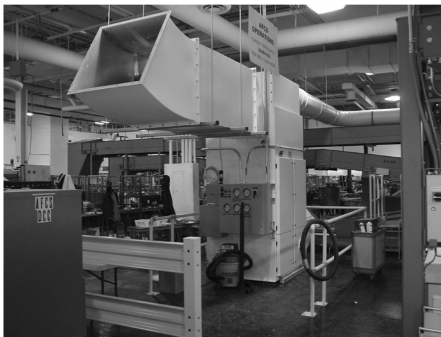
FIGURE 7. Part of the ventilation and filtration system installed on a USPS 010 Culling System. The white filter/fan housing is the 8000 cfm (3.8 m 3 /sec) unit (Unit A-Floor) tested as part of this study.
