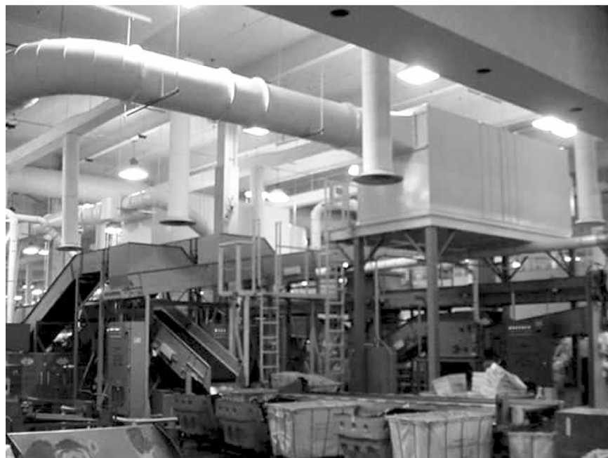
FIGURE 1. Part of the ventilation and filtration system installed on a USPS 010 Culling System. The large white filter/fan housing (upper right) was one of the 18,000 cfm ( 8.5 \text{ m}^3/\text{sec} ) units tested as part of this study.
