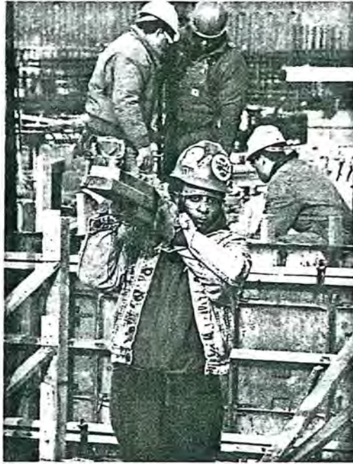
FIG. 42-1. Construction workers building a large sewage treatment plant. Women remain a small minority of the construction workforce in most countries. (Photograph by Marvin Lewiton.)
