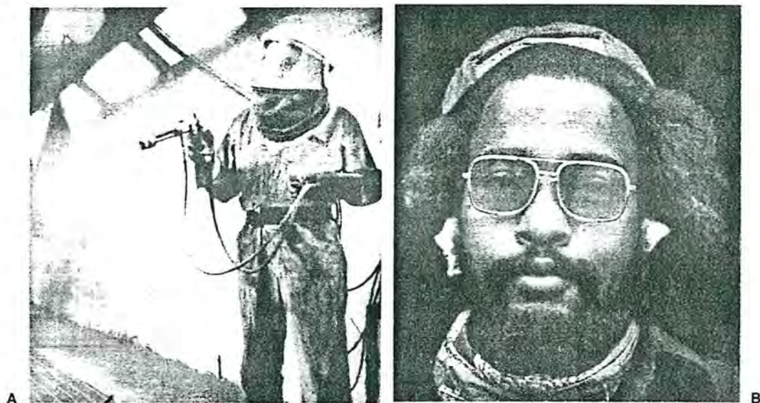
FIGURE 7-6 • (A) Spray painter with respiratory protection. (B) Makeshift PPE. Cotton plugs are not effective as PPE; only adequately fitting earplugs or earmuffs are effective. (Photographs by Earl Dotter.)
