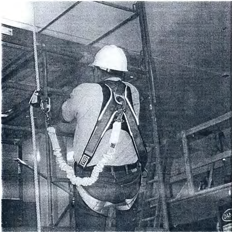
FIGURE 22-5 • Worker wearing a full-body harness with attached lanyard (Photograph courtesy of the Construction Safety Council.)
