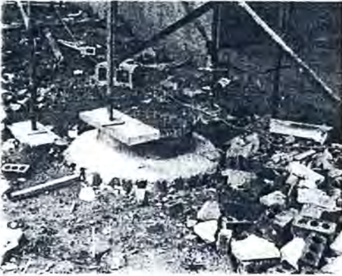
FIGURE 22-2 • Example of poor housekeeping on a construction site. Loose bricks, lumber, and other debris create a potential tripping hazard for workers.
