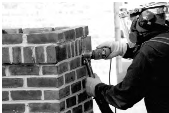
FIGURE 3 Ventilated mortar rake in operation.
