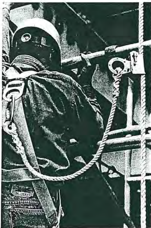
FIG. 24-5. Ironworker using a full-body harness and lanyard attached to a rope grab. This worker has the flexibility to move up the structure while maintaining fall protection. (Photograph courtesy of the Construction Safety Council.)
