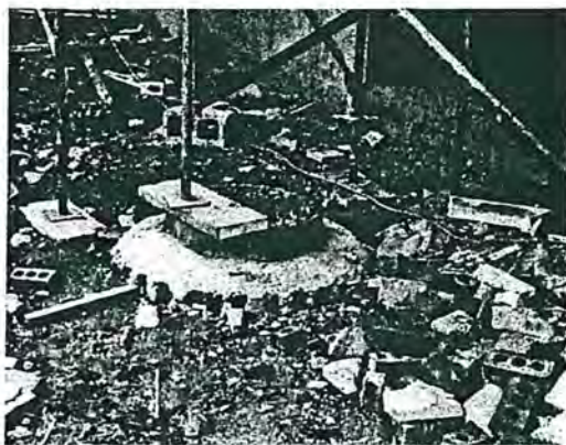
FIG. 24-2. Example of poor housekeeping on a construction site. Loose bricks, lumber, and other debris create a potential tripping hazard for workers.
