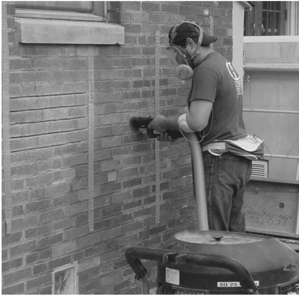
(B) Mortar removal with dust control
