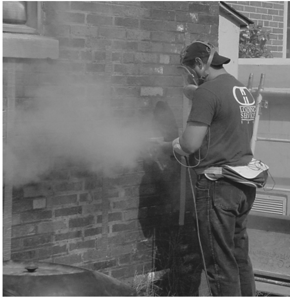
(A) Mortar removal without dust control
