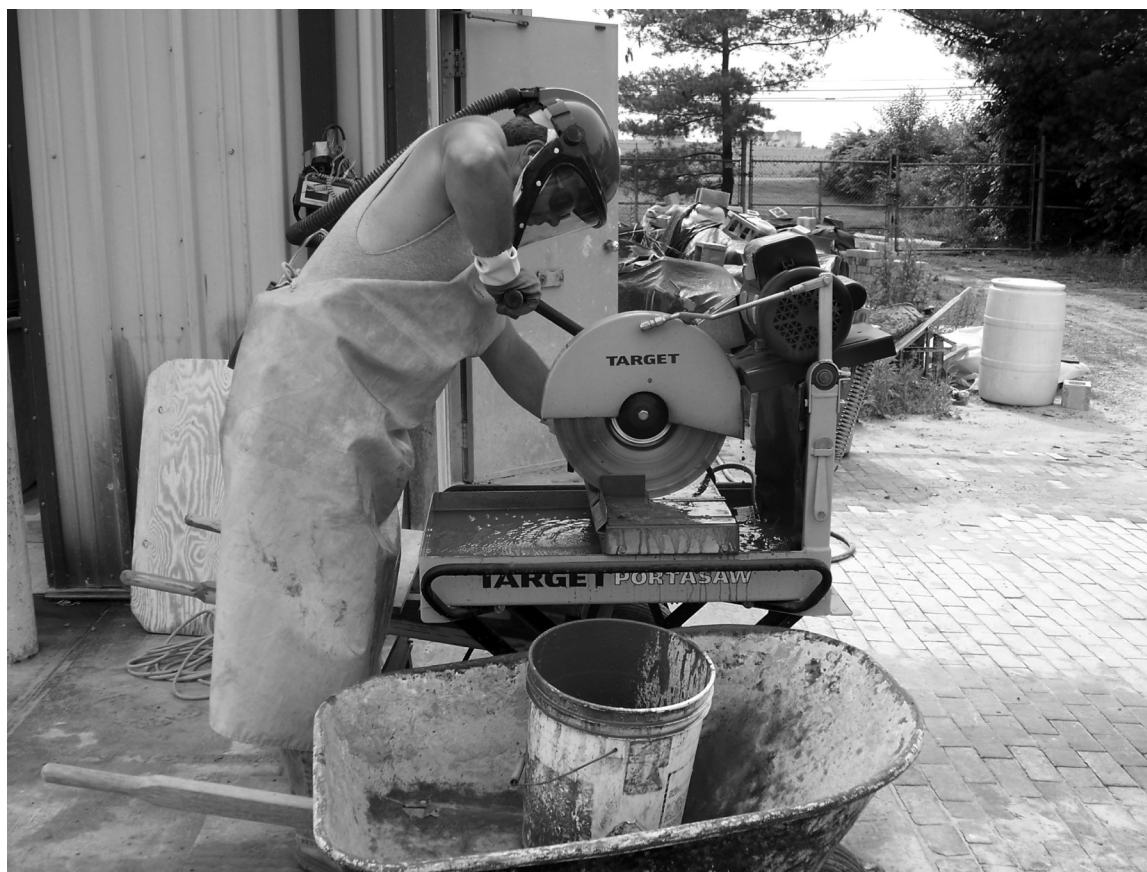
Photo 3. Brick cutting using Target® stationary wet saw
