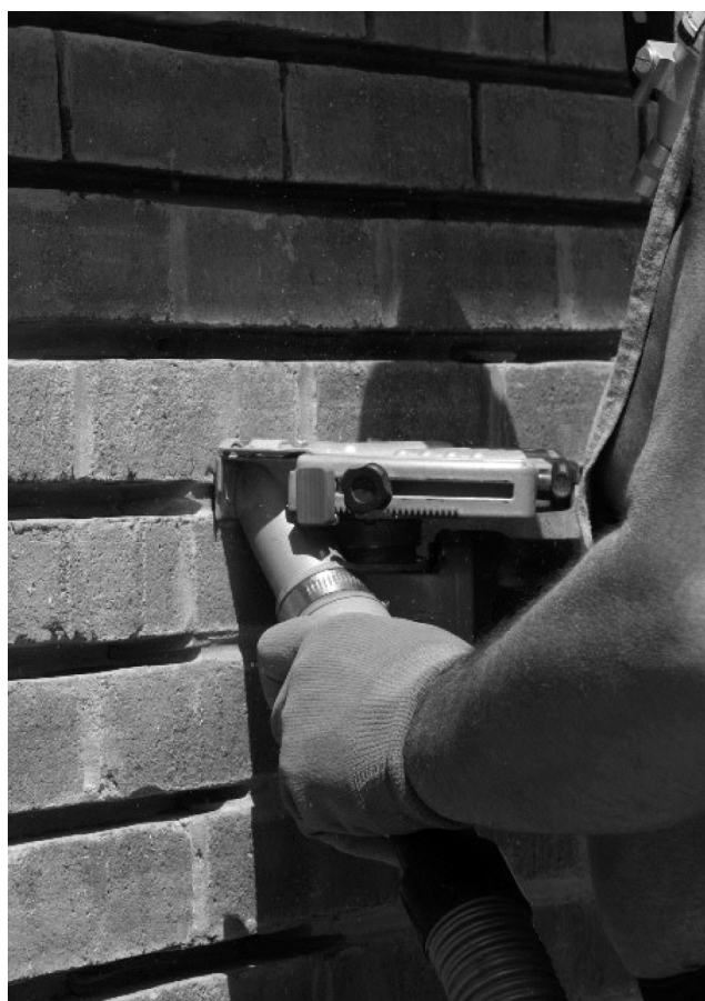
Photo 4. Tuckpointing using Bosch® grinder
