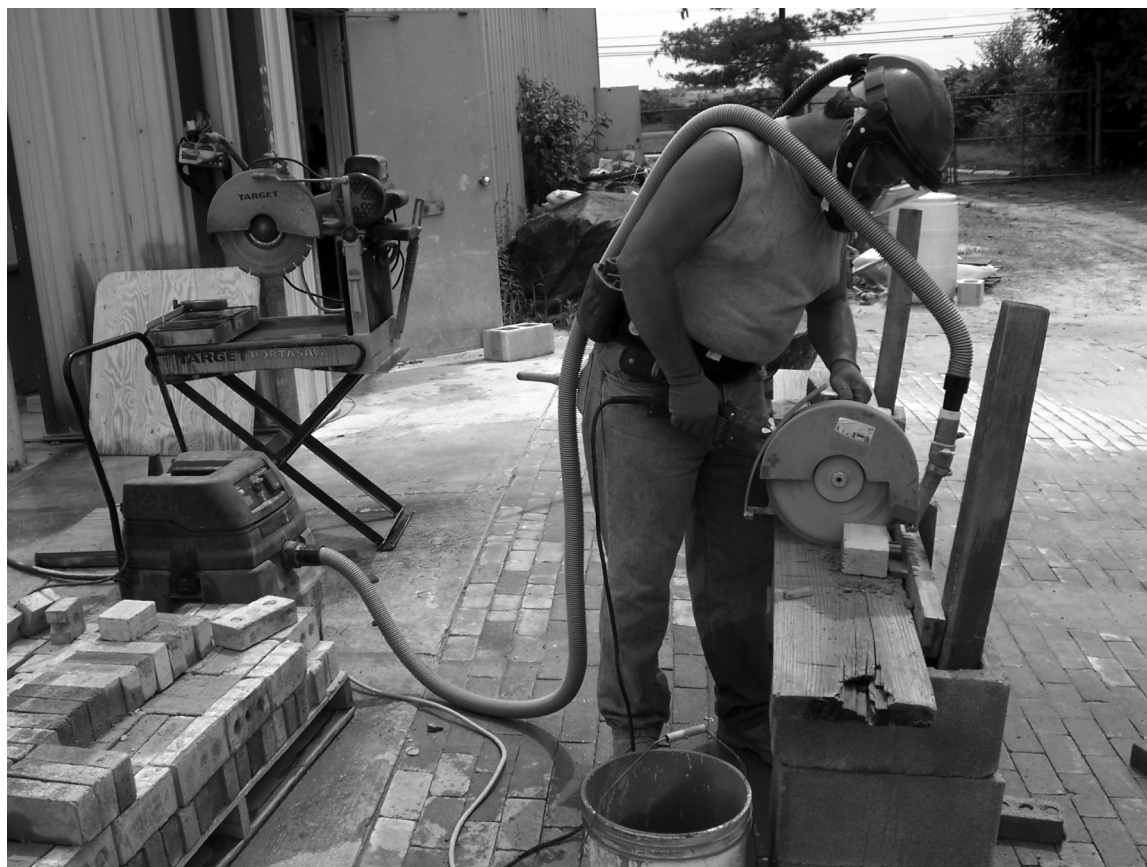
Photo 1. Block cutting using Bosch® abrasive cutter with Bosch Airsweep™ vacuum
