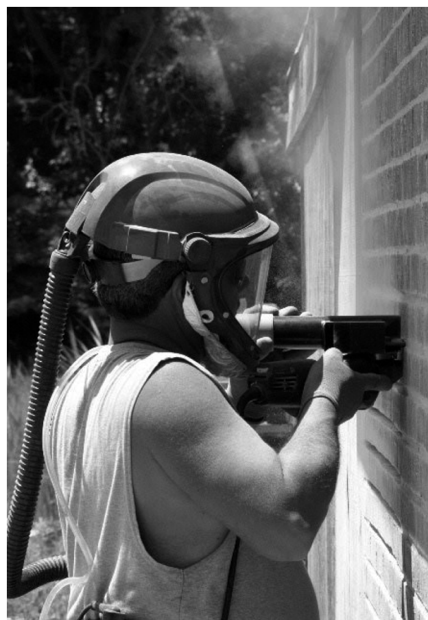
Photo 5. Tuckpointing using Metabo® grinder with Dust Director® shroud
