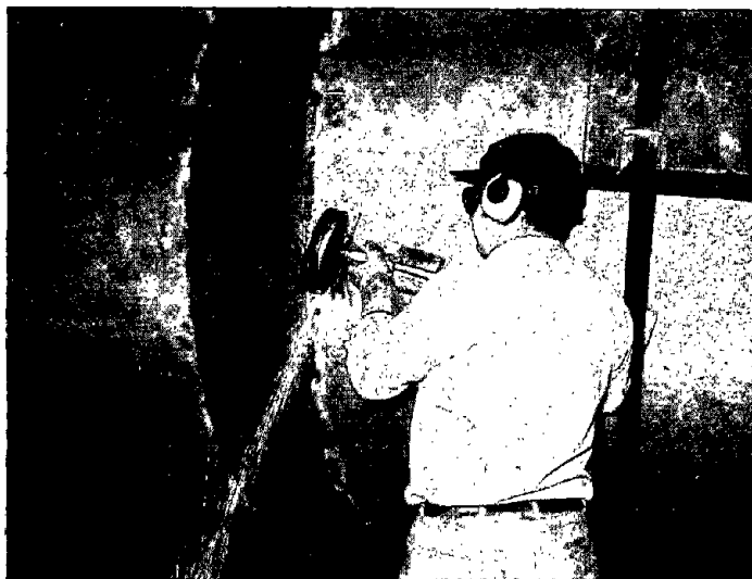
Figure 1-7. Employee Grinding on Boiler Drum, Bay 11, Boiler Plant (95 dBA)
