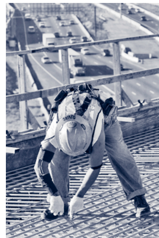
FIGURE 3. Construction worker being evaluated by engineers for musculoskeletal disorder risk factors
