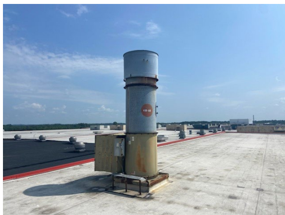
Figure B1. Exhaust stack for the 4-roll local exhaust ventilation system. Photo by NIOSH.
