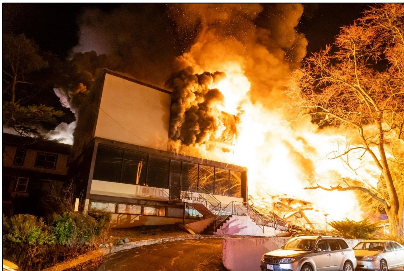
Photo 8. The cantilever collapse of Side Bravo/Side Charlie corner of the original building. The time was approximately 02:08 hours. (Photo Courtesy of Kenneth Flynn)
