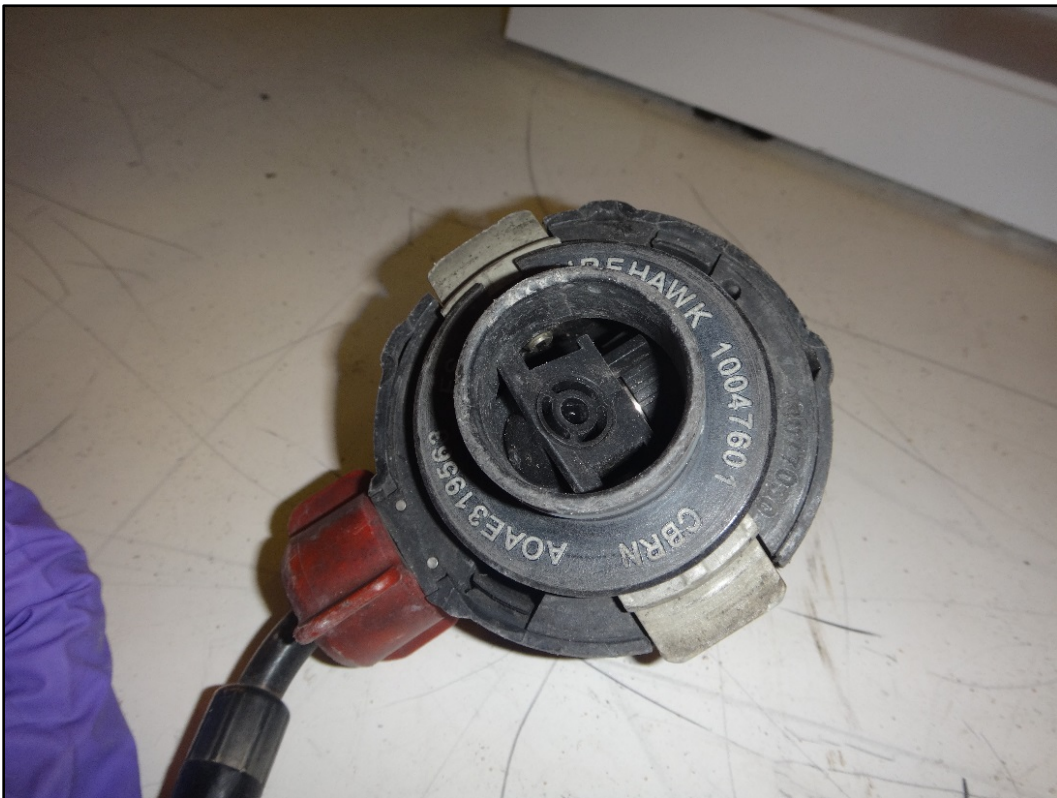
Figure 6: Inside flange, MMR
