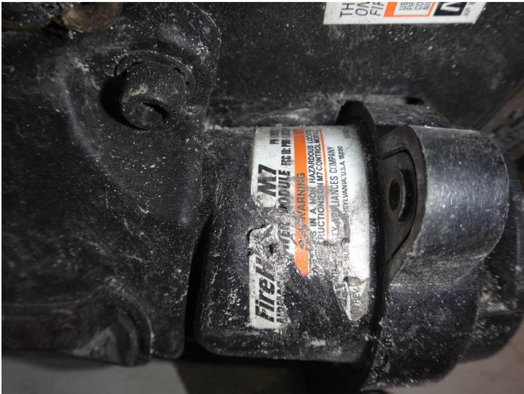
Figure 23: Damaged label on PASS control module
