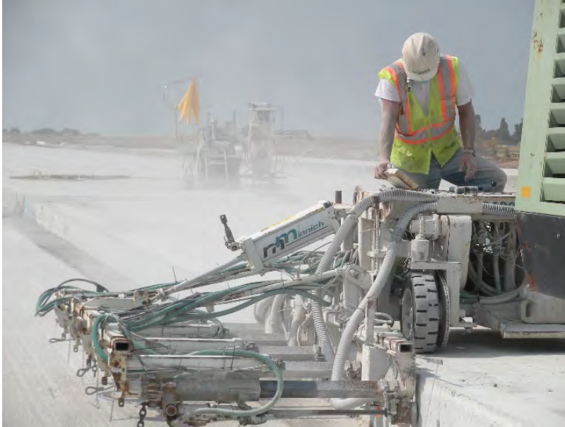
Figure 5. Worker performing dowel drilling on a concrete slab.
