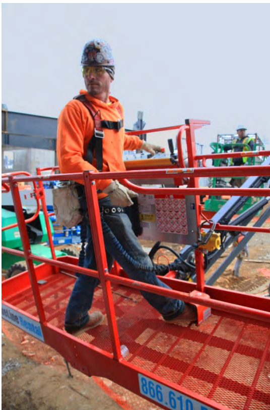
Figure 65. A NIOSH study showed that fall arrest systems on aerial lifts offer effective fall protection. [Credit Turner Construction/Earl Dotter/CPWR]
