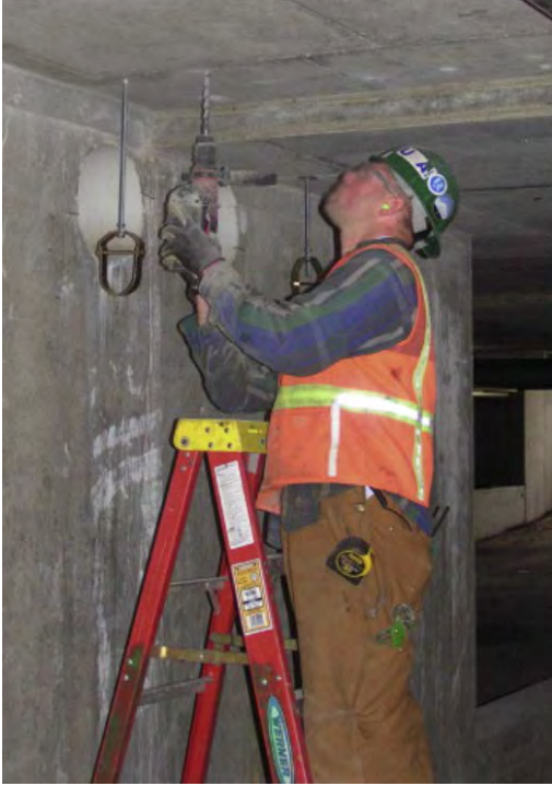
Figure 26. Construction worker performing traditional overhead drilling.
