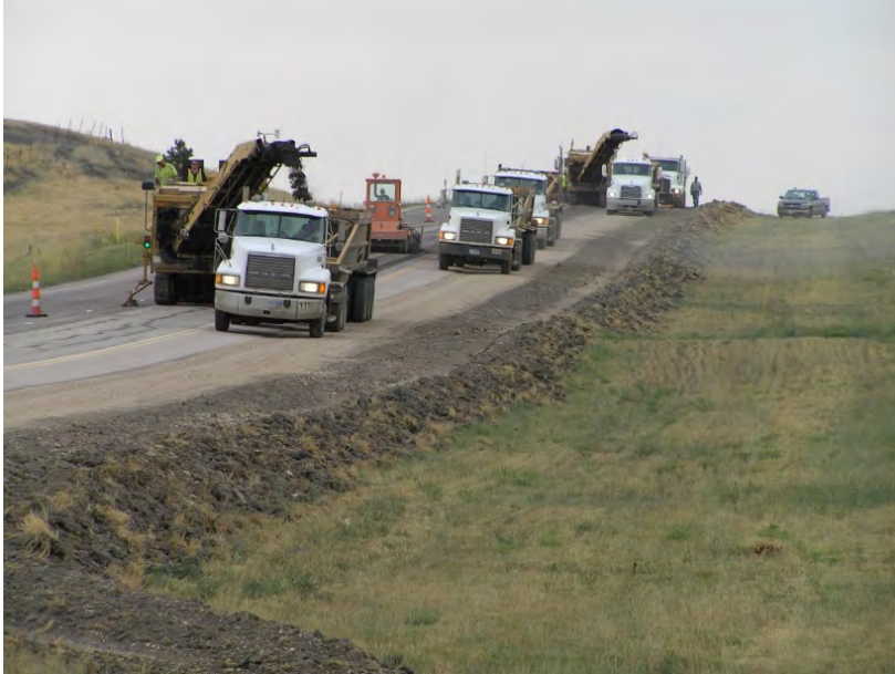
Figure 7. Asphalt milling machines in use during road construction.
