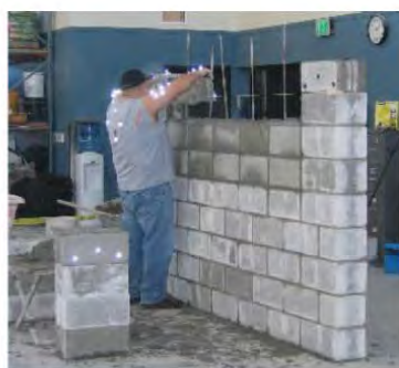
(a) Placing conventional CMU
