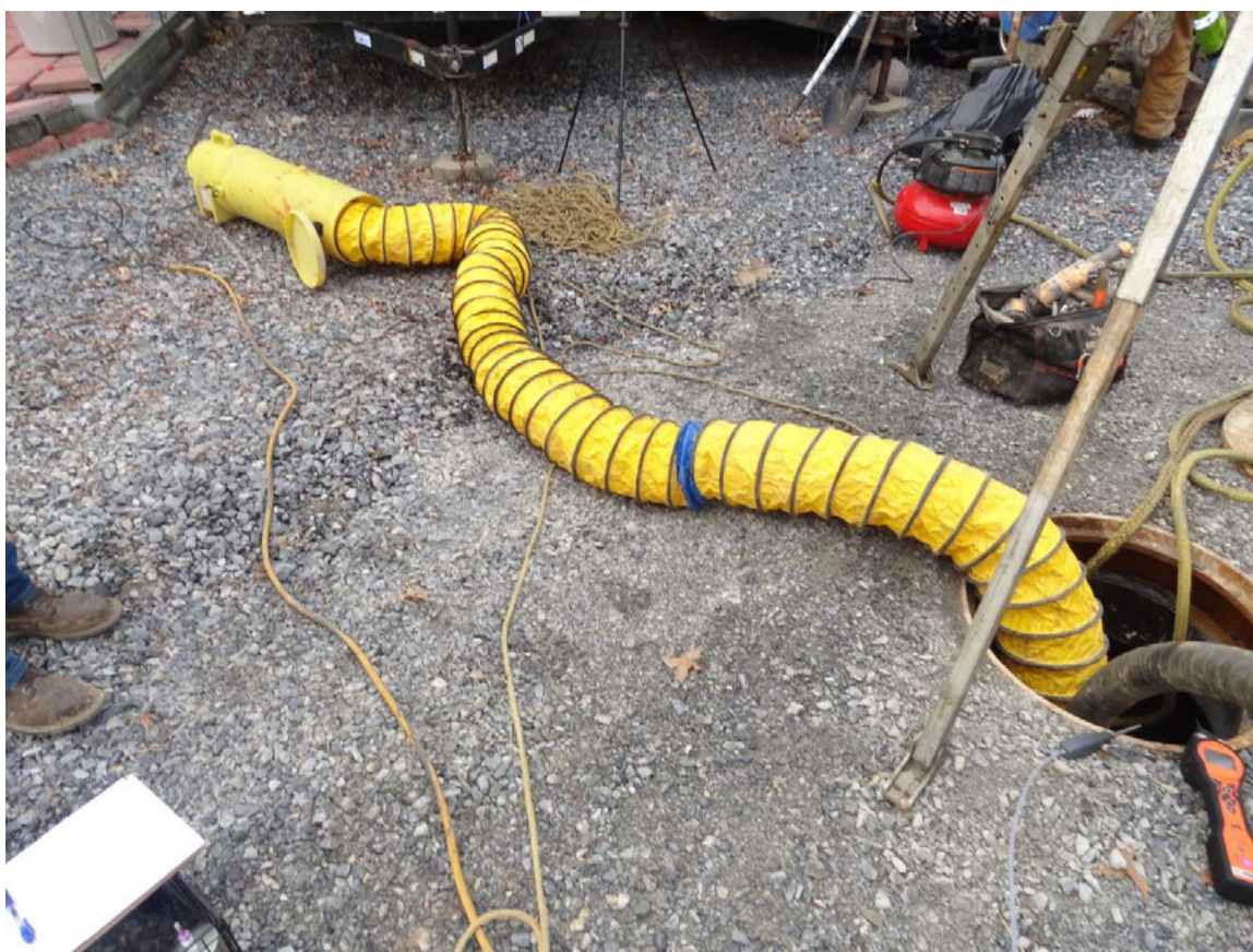
Figure 2. Manhole ventilation blower used to provide dilution ventilation to manhole during CIPP installation tasks, February 6, 2018.
